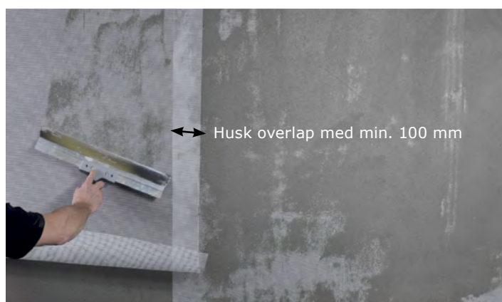
Overlap med minimum 100 mm
