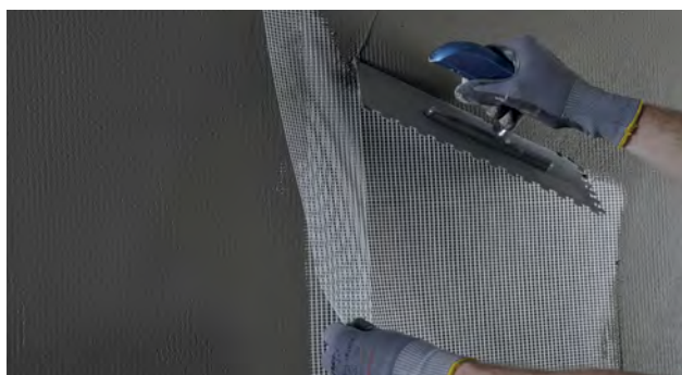
Montering af net med min. 10 cm overlap
