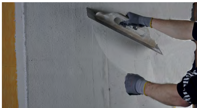
Montering af net med min. 10 cm overlap
