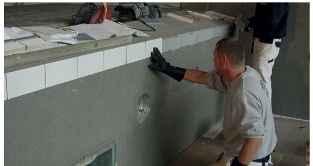
Fixing tiles onto the moist adhesive
