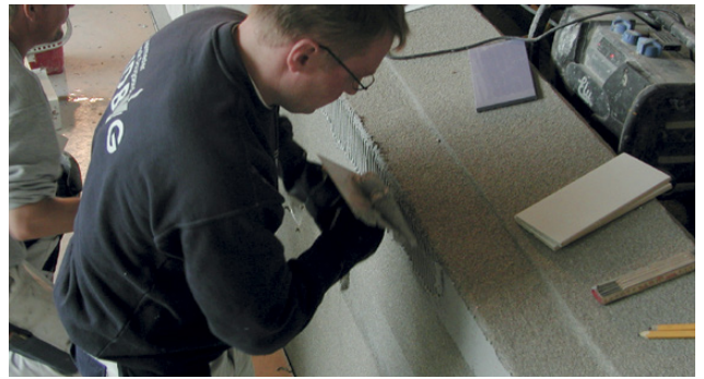
Applying Alfix C2 Epoxy with notched trowel
