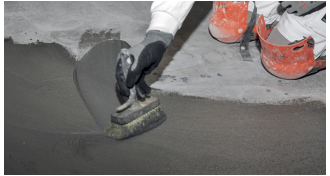
Slurry bonding with a brush
