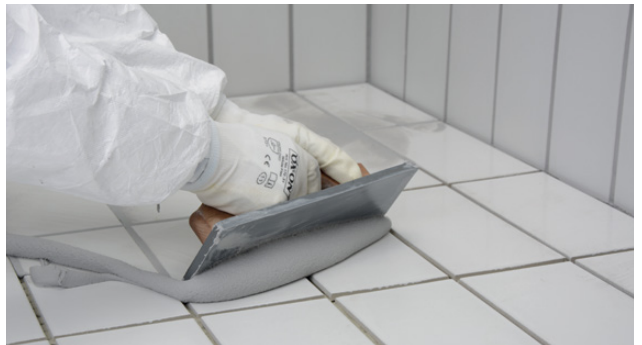
Applying to floor with epoxy grouting float
