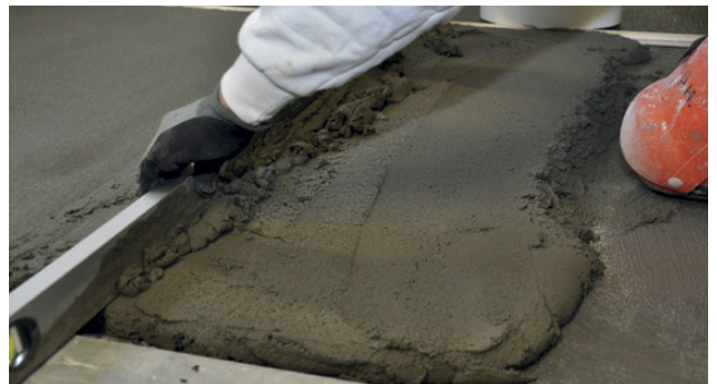
Levelling off with a straight edge
