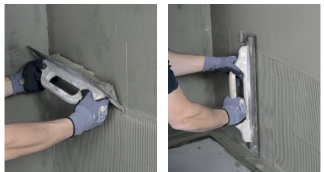
Applying 2K Sealing membrane and smoothing
