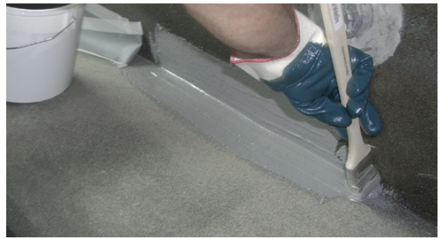
Applying Alfix Epoxy Membrane
