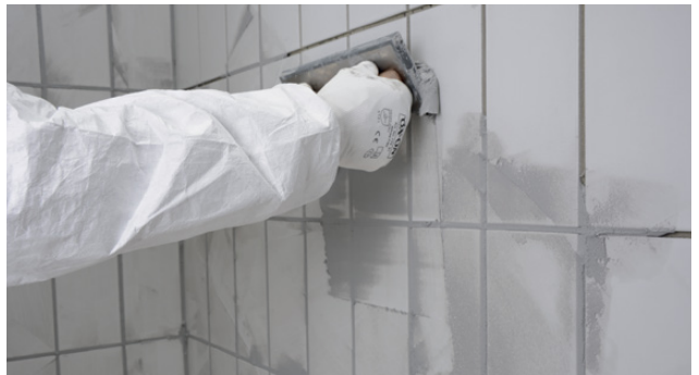
Applying to wall with epoxy grouting float
