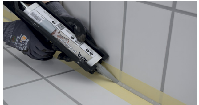
When the primer is dry, fill-in Alfix M-Silicon
