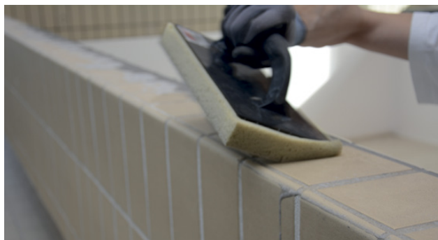
Adjust joints to match the tile design
