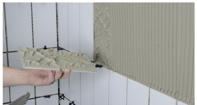
Checking adhesive coverage
