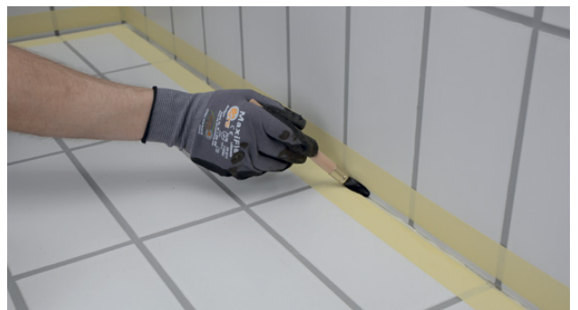
Priming after applying masking tape
