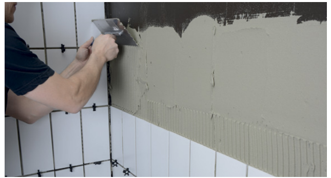
Applying tile adhesive with a notched trowel
