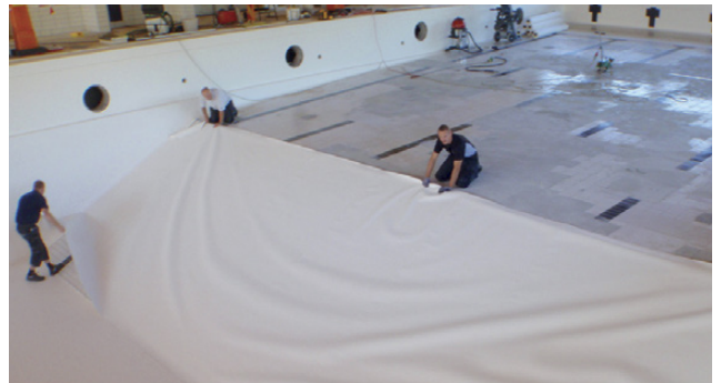
Installing PVC liner
