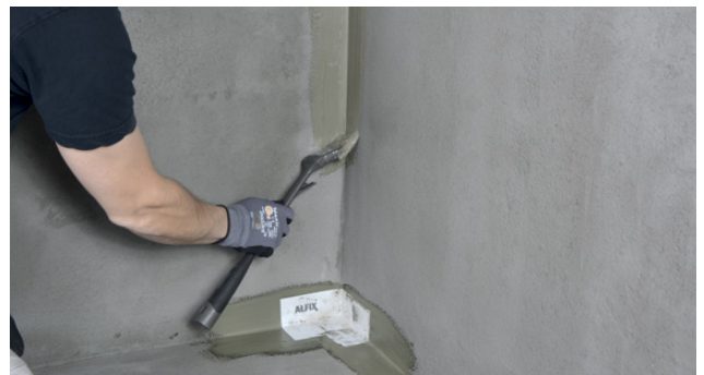
Bedding Alfix VT corner in sealing membrane
