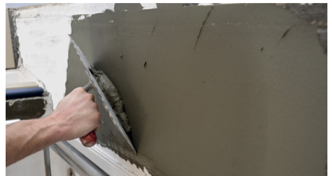
Applying contact coat
