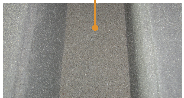
Surface saturated with sand
