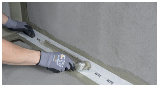
Bedding Alfix VT strip in sealing membrane
