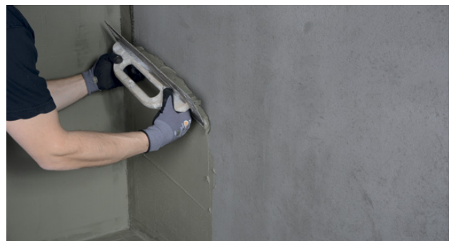
Applying Alfix 2K Sealing membrane – pore filling coat
