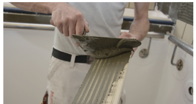
Back buttering the tile with a thin coat of adhesive
