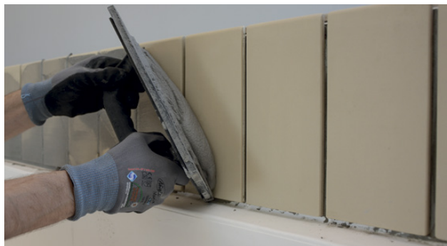
Applying Alfix IndustryFuge CeraFill 18
