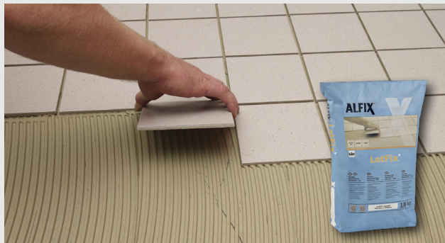
Flismontering i Alfix flislim
